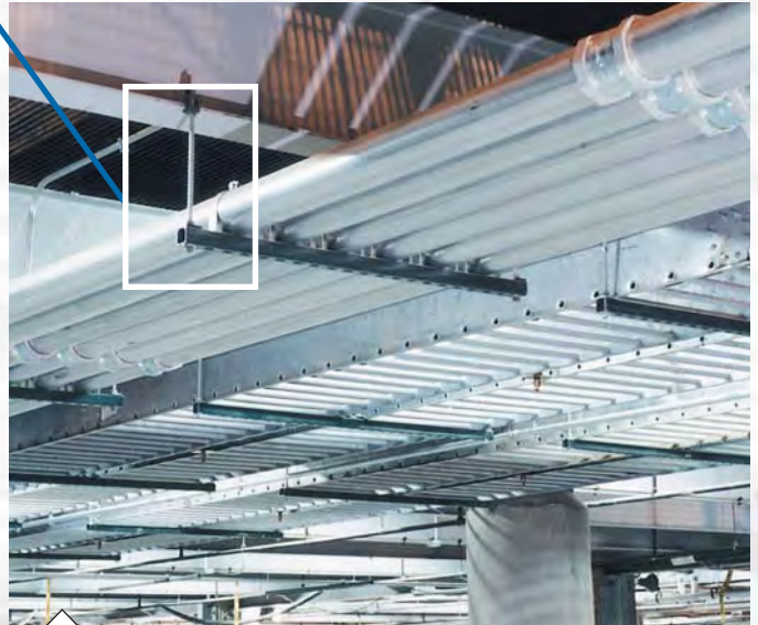
Beam clamp accepts standard threaded rod.
